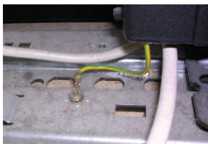
Fig.50. Grounding connection of a fridge.
